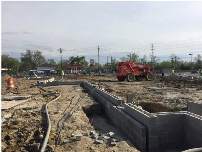
Project Site on May 7, 2019 View of the Exterior Foundation Wall.
