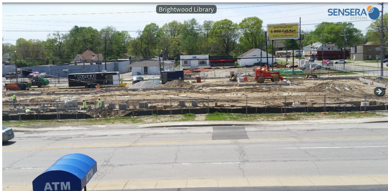
Project Site on May 6, 2019
