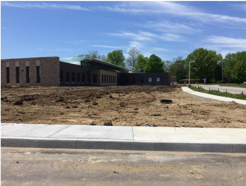
Project Site on May 6, 2019 View of the Building From the East.
